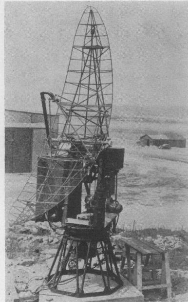
Fig. 3—Fanned-beam antenna.
